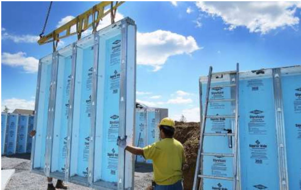
Figure 2: Precast Concrete Foundations Installed in a Day with Cranes
