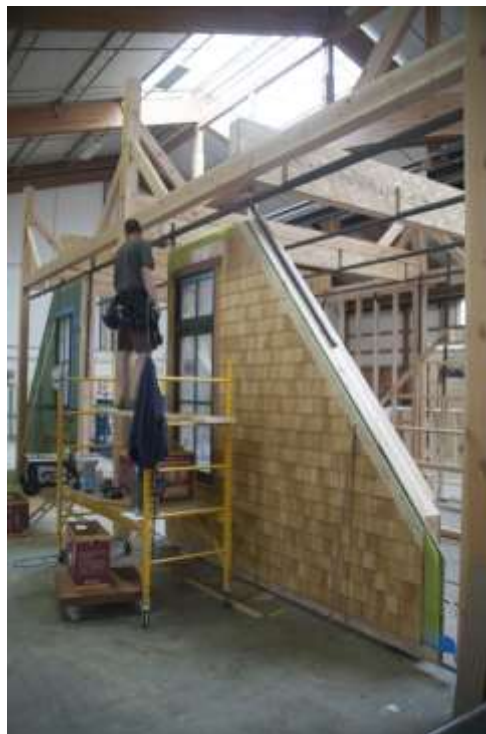
Figure 3: Unity Homes wall panel production
