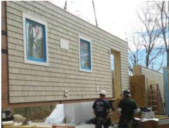
Figure 5: Unity Homes field assembly
